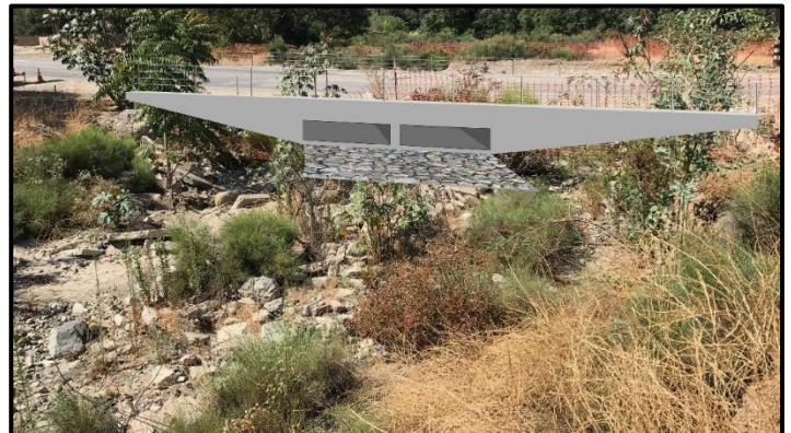
VISUALIZATION: The box culvert will allow Coldwater Creek to flow under Temescal Canyon Road . Not pictured, the culvert will have a guard rail. The $335,000 construction cost is low because the county provided the concrete boxes needed for the project.
