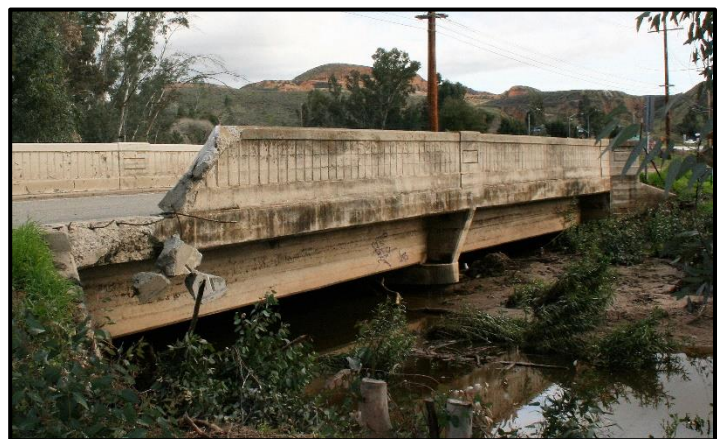
ROAD CLOSURE: Recent rains damaged the Temescal Canyon Road bridge north of Lake Street. The road is closed until repairs can be made.
